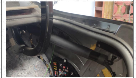
8. Install our electric pole ("L" left "R" right)
